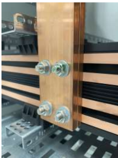
Example of connection up to 1600 A
